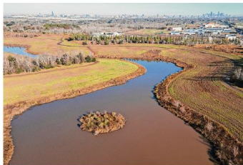
The 100-acre green space will emerge from a detention basin owned by the Harris County Flood Control District. Hill continues on A6
